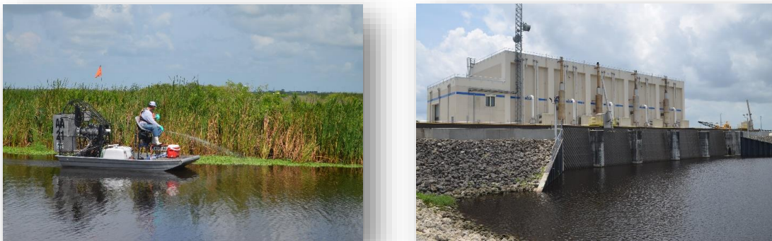
Aquatic plant management contractor controlling invasive water lettuce in a canal (left) upstream of the water pumping station (right) that regulates water flow from agricultural areas before entering the STA and water conservation areas. Water lettuce is frequently managed throughout the year along the canal banks to prevent plant jams in the downstream water control structure.
